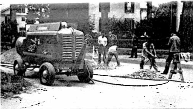
Portable compressor on road repair service
