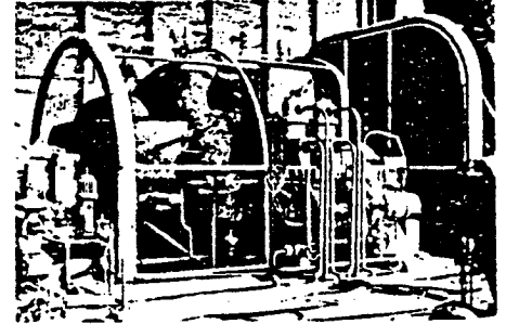
High Temperature Industrial Thermal Insulation —Because of its low thermal conductivity, coupled with the ease with which it accommodates itself to irregular surfaces, SPRAYED "LIMPET" ASBESTOS has been proved to be one of the most efficient forms of insulation.
