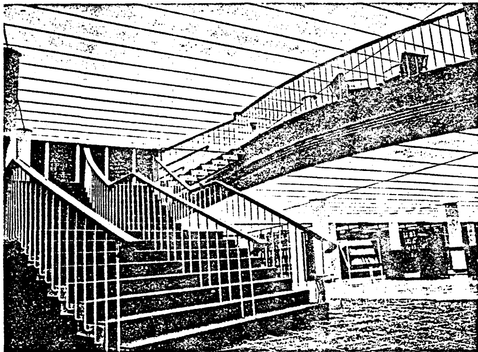
READING & EXHIBITION ROOM - Charlotte Public Library, Charlotte, N.C. Sound reduction. Applied to slab above suspended luminous ceiling. Applicator: C.W. Kirkland Co., Charlotte, N.C.
