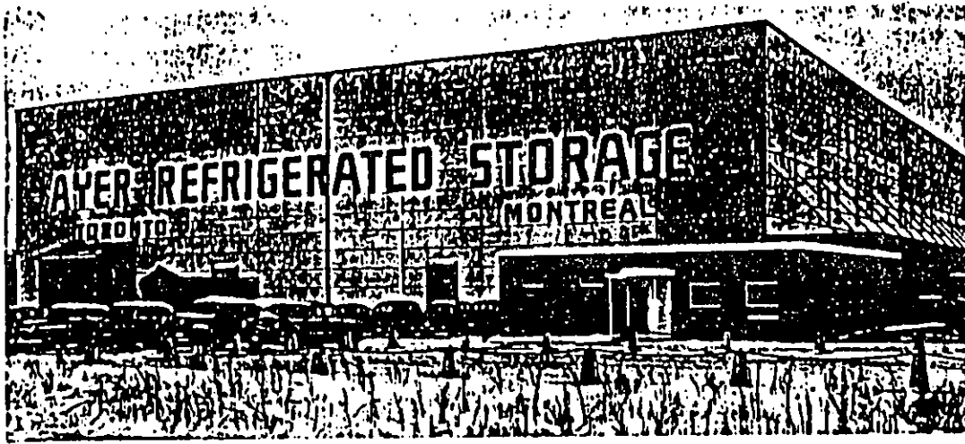
Ayer Refrigerated Storage Limited at Toronto, Ontario.
