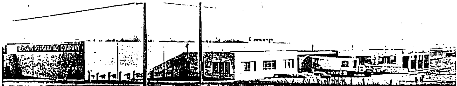
Merchants Refrigerating Company at Hopkins, Minnesota.
