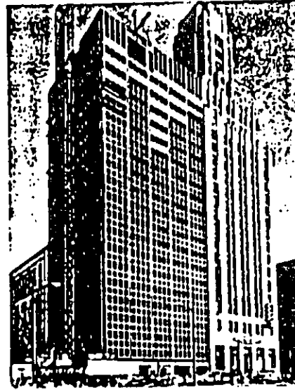
Tishman Building in Buffalo, New York.
